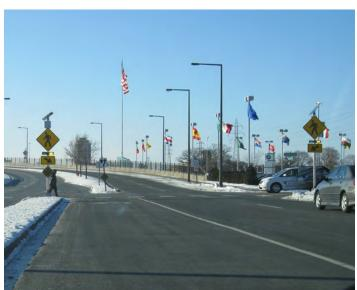
Mid-block crossing with pedestrian-activated flashing lights and median island
