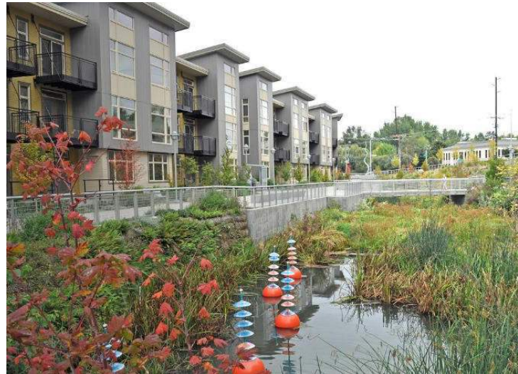
Attractive green stormwater facility with adjacent path v
