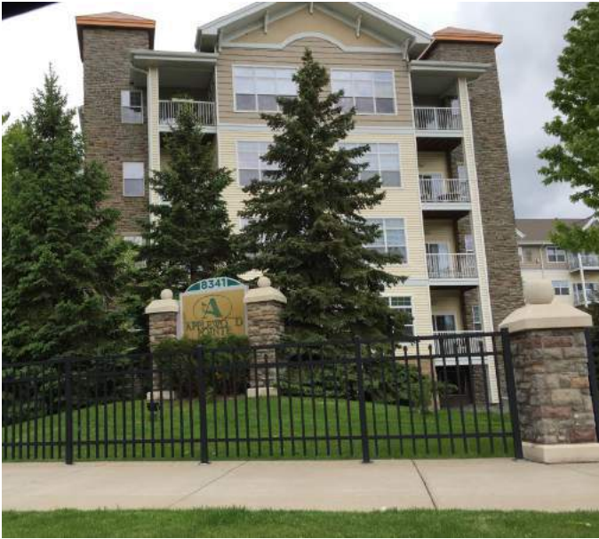
This multi-family building is typical of housing on Lyndale Avenue
