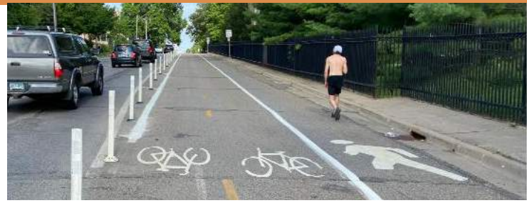
Multi-modal path replaced one traffic lane using low cost bollards ^
