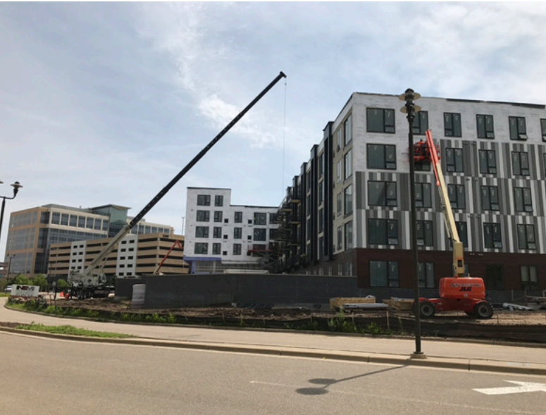
A 179 unit apartment building under construction.
