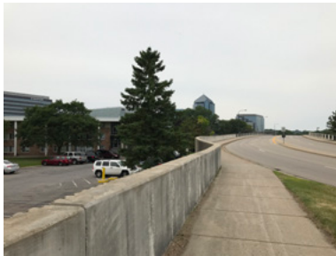
Bridge looking west over Normandale Boulevard.
