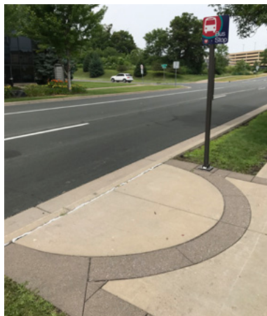
Decorative concrete pad
