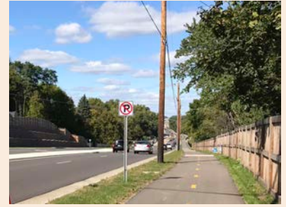
Segments of the multi-use trail along Normandale Boulevard were reconstructed in 2018.
