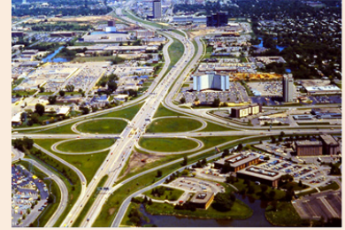
The first phase of the I35W/I494 interchange reconstruction is expected to begin in 2022.
