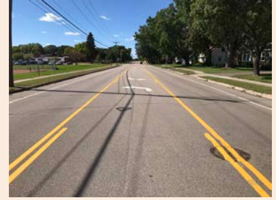
Conversion of 4-lane road to 3-lane road with bike lanes in shoulder.
