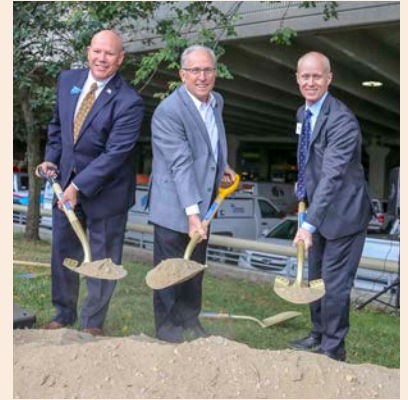
Mall of America transit station renovations began in 2018 with completion expected in late 2019.
