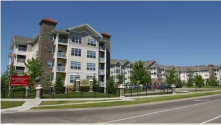
Applewood Pointe Lyndale, Senior Cooperative: Built 2005, 95 units, 25 units/acre. Previous use: Retail.
