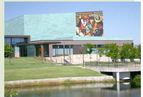
Bloomington Civic Plaza houses City Hall, Police and the Arts Center and has been a focal point for building and renewing the community.
