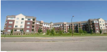
Realife Lyndale, Senior Cooperative: Built 2003, 96 units, 23 units/acre. Previous use: Lumberyard.
