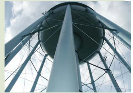
Valley View Water Tower
