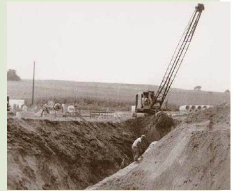
Sewer pipe installation, 1960.
